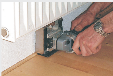
Cutting expansion joints under radiators
